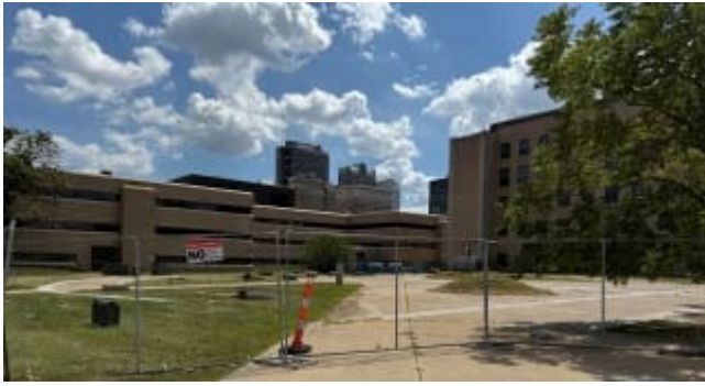
View of subject site
