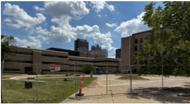
View of subject site
