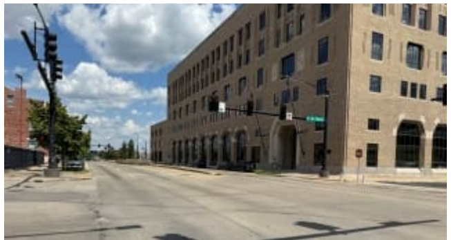
View of Tucker Blvd facing north
