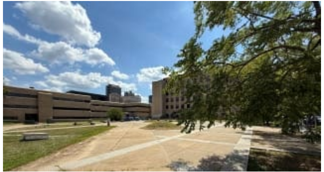
View of subject site
