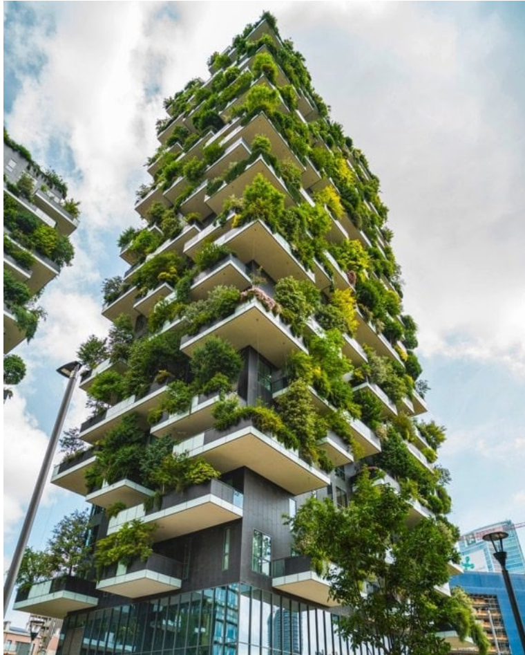
Figure 44 – Vegetation Throughout the Façade
