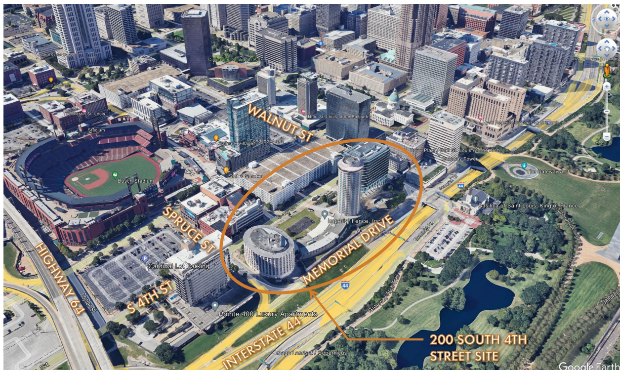
Figure 6 – Aerial Looking Northwest
