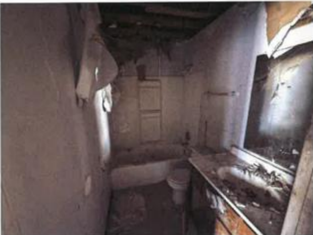
166. Building No. 17 – View of 3825 McRee Avenue bathroom.
