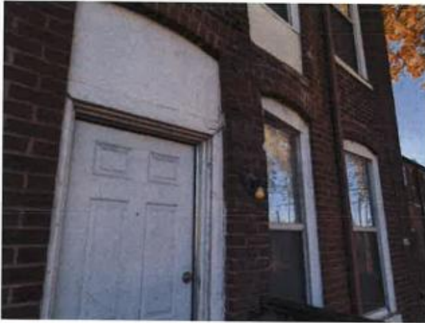
187. Building No. 21 – View of bowed brick wall at the north side of the building.
