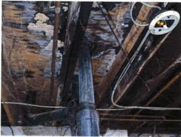
177. Building No. 19 – View of moisture damaged wood joists and decking at 3840 McRee Avenue.
