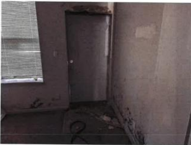
170. Building No. 18 – View of damaged finishes and door hardware, as well as organic growth in 3837A McRee Avenue.
