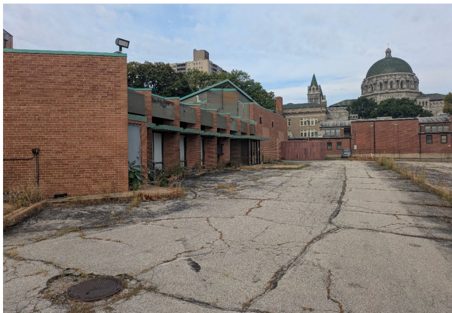
Rear/North façade and parking lot conditions
