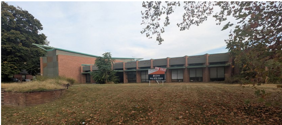
Southern façade view from Lindell ROW
