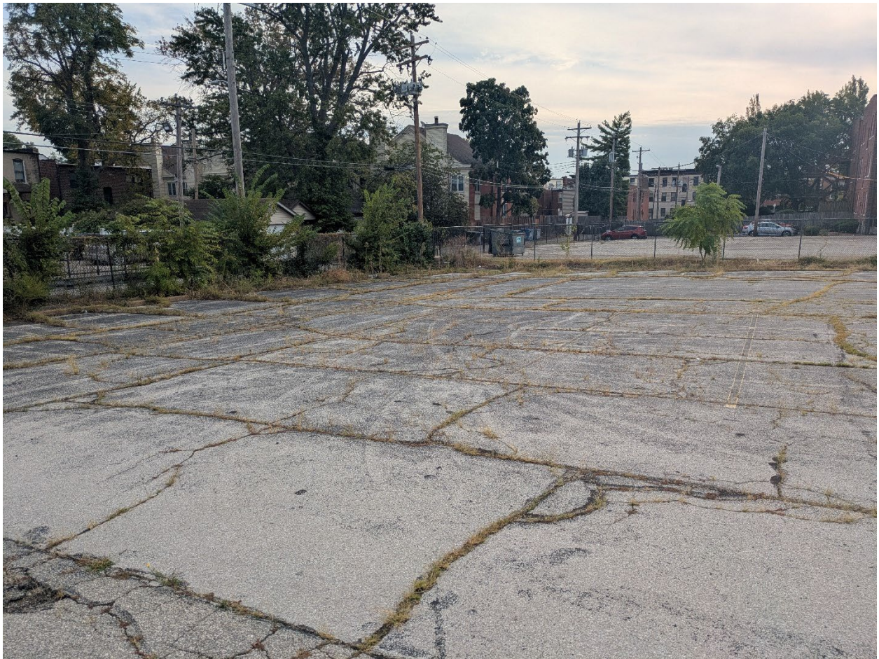
Figure 3 – Parking lot conditions.
