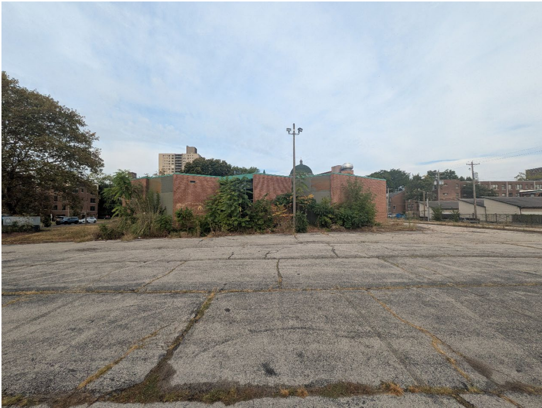
Figure 4 – East façade of the building and parking lot conditions.
