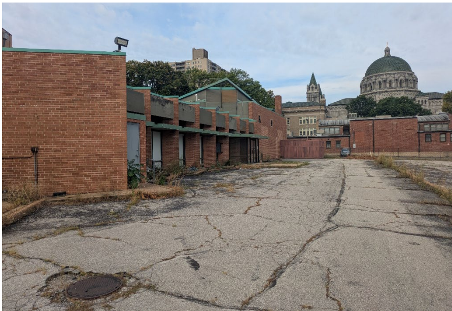
Rear/North façade and parking lot conditions
