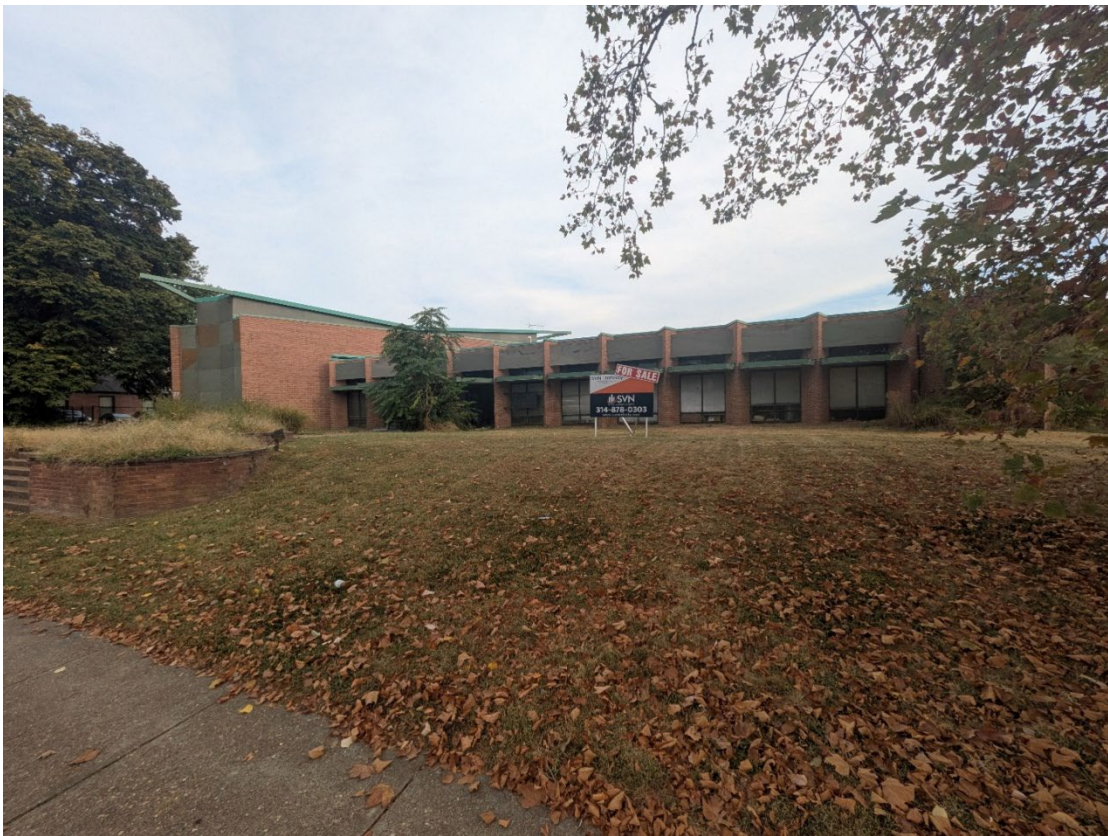
Figure 5 – South façade of the building looking north from Lindell Boulevard.
